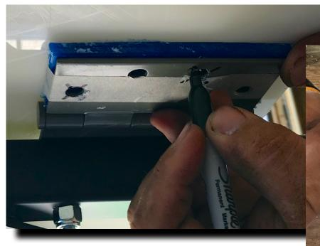
mark the holes, remove the seat, and drill,
